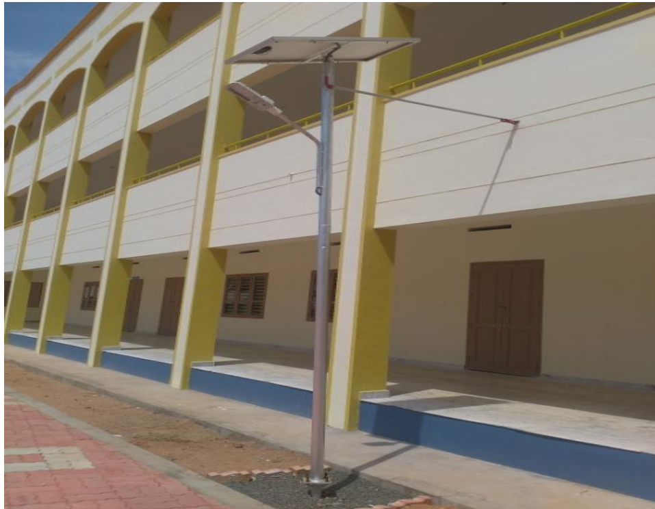
Solar Lighting system
