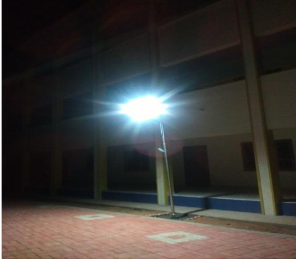
Solar Lighting system - Working condition
